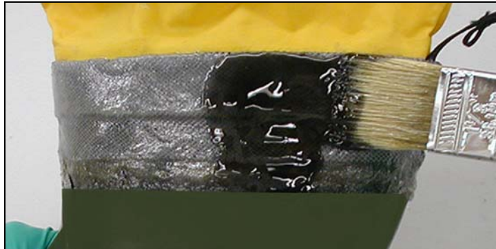
Figure 22. Step n. Boot Replacement
